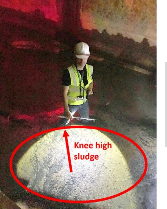
A properly maintained storm water sump pit should be clean, free of sludge, silt and debris, and empty in anticipation of the next storm so that it can do its job.
